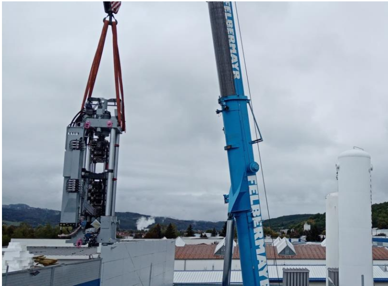
SACMI 300t press unloader (left), press after successful installation (right)
